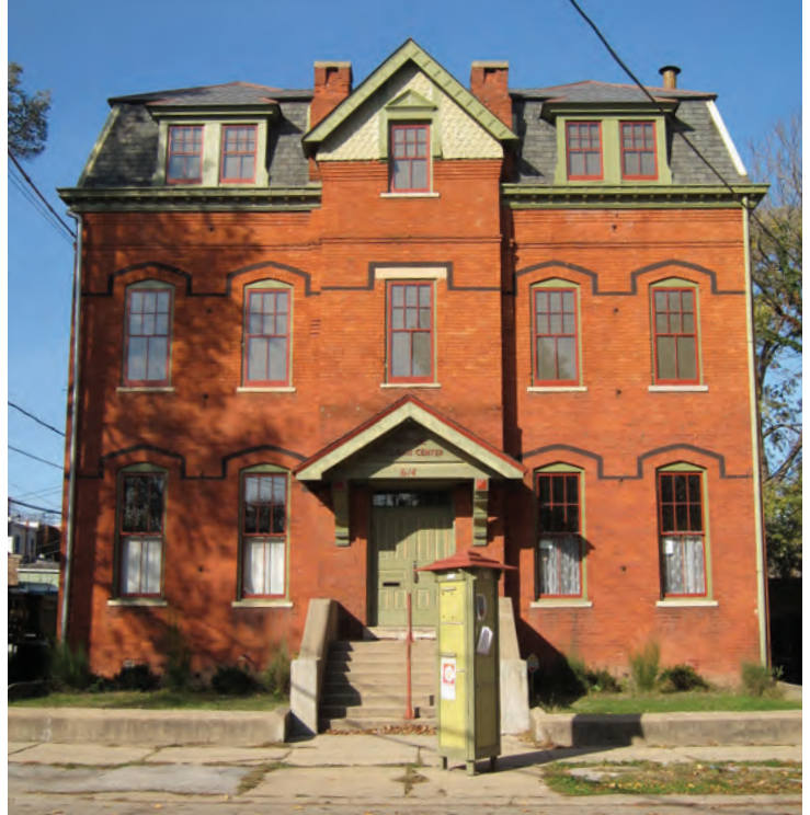
Top: Market Hall, 2012. Middle: Aerial view of Market Hall Bottom: Masonic Hall (Historic Pullman Center), 2012.
