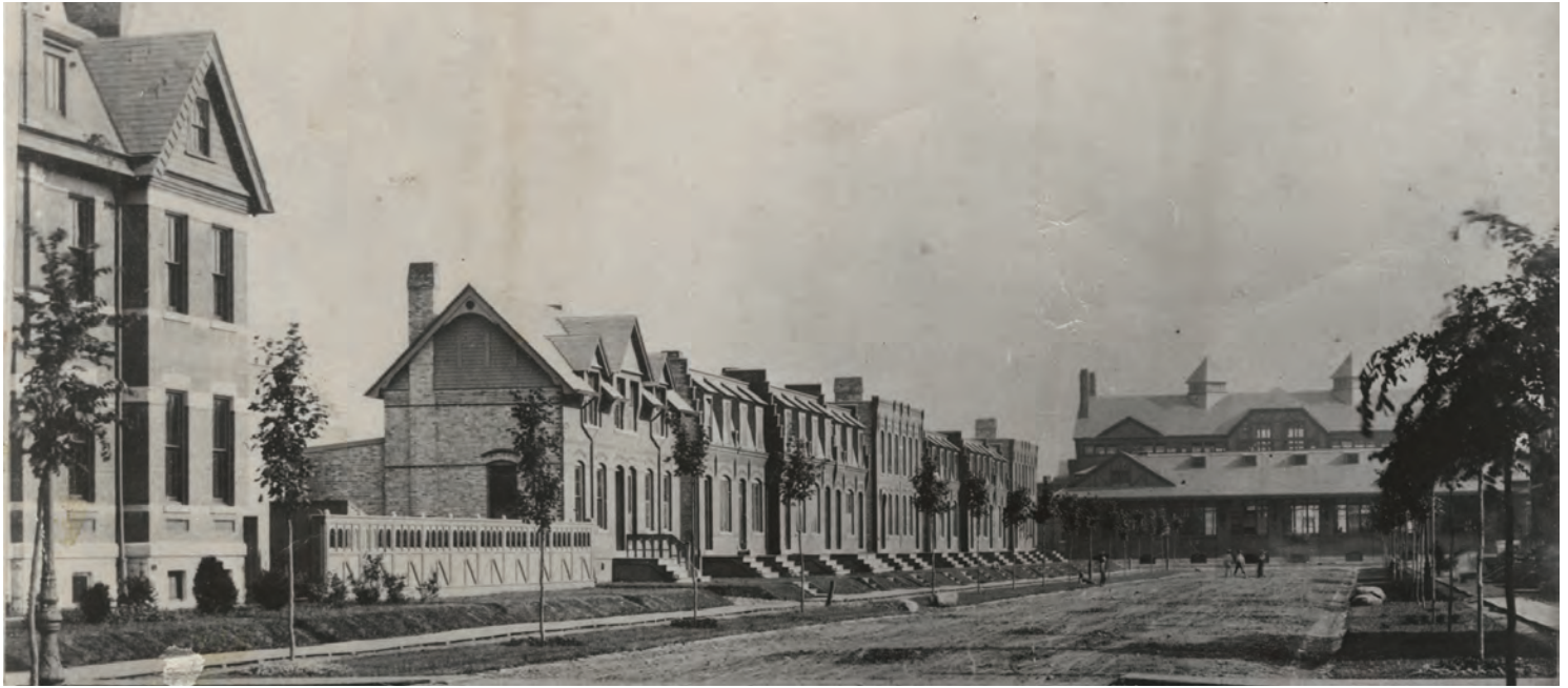
View of east side of 11100 block of Champlain Avenue with the original Market Hall in the distance, c.1883. Courtesy of the Industrial Heritage Archives at Pullman State Historic Site.
