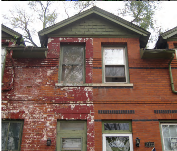
Top: Houses rehabilitated by CNI in North Pullman. Middle: An ongoing CNI Rehabilitation in North Pullman. Bottom: Detail of houses in South Pullman.
