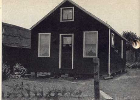
A keen desire coupled with determined perseverance has produced a home of which any man would be proud. The hedge shown in the foreground was grown from seed.
