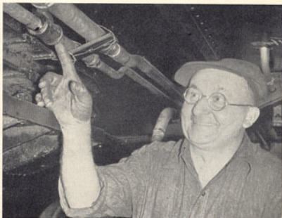
The new style threaded T that is simple and light. It is plenty strong enough.
